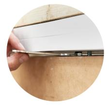
**15. Lock Hangers** Tighten off the Hanger lock-bolts with the spanner provided.
