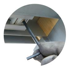
**16. Adjust Stops** Adjust the stops inside the track to ensure the doors is stopped in the correct position.
