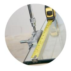
Fix the gear brackets 80mm from edge of the doors.
