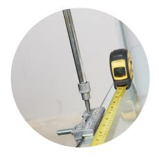
Fit the clamps 150mm from the edge of the leaf to the centre of the clamp.
