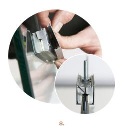
Fit the cover plates by hooking them on the top and pressing down until they click into the place against the glass. Ensure the door leaf is installed and hung before fitting the cover plates to allow any adjustment.
