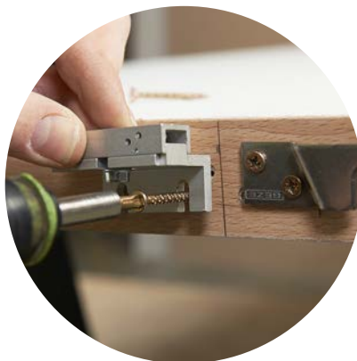
2. Fix the carrier Brackets onto the Door leaf 190mm from the back edge of the Doors.
