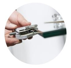
STEP 5 Place the clamps on the glass leaf and tighten the bolts.
