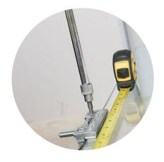
STEP 6 Fit the clamps 150mm from the edge of the leaf to the centre of the clamp.
